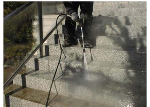
Efflo removal is carried out with a high-pressure washing machine.
