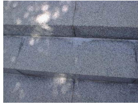
efflo is flowing out from the crack.
