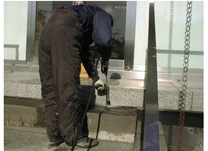
Efflo removal is carried out with a high-pressure washing machine.
