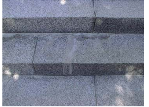
efflo is flowing out from the crack.
