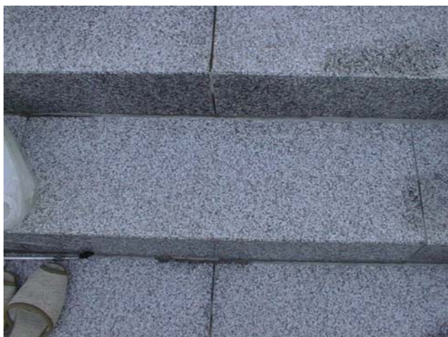
Hydroproof The completion of construction
