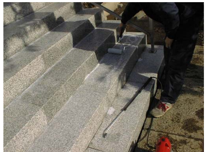
Waterproofing protection processing construction process
