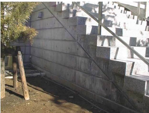
RC side wall after Efflorescence processing
