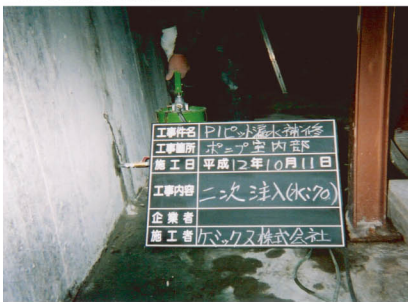
Water leak prevention work (blast-furnace slag injection) in underground pit
