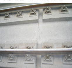
Penetration crack developed at the railway track basement floor slab
