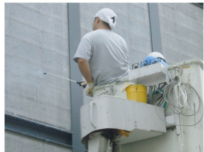
waterproofing work at brick joints
