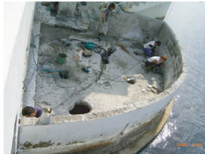
swimming pool improvement work at Kitahara residence in Sashima
